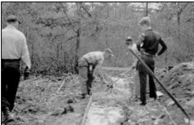
1950's firm foundation for the Octoraro 22 lodge
