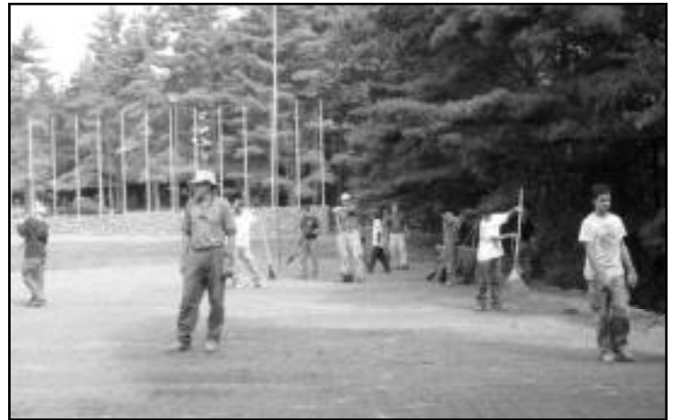
Leveled and being readied for seed and straw
