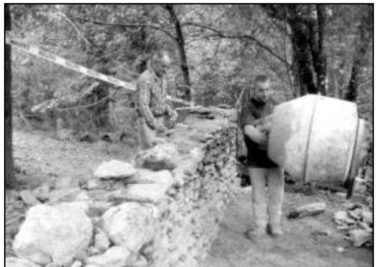
Stonewall construction at end of field
