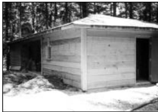
Newly erected C.O.P.E. building readies for camp program
