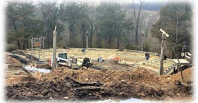
Anyone who has sat in the visitor section of the circle may know the benches tilted forward due to hydrostatic pressure. This project addresses that problem by diverting water away from the seating area and using the large boulders and concrete to hold the ground and seats in place. While the heavy work is being handled by a landscaping company, Horseshoe volunteers are needed to help with the drainage, seeding, plus bringing electric and plumbing to the site.
