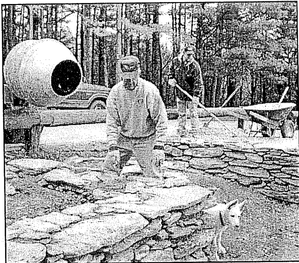
Construction Workers Building Head Wall
