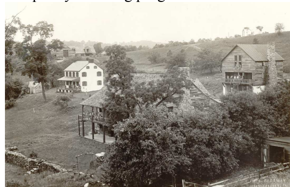
View of White House HQ, Kindness Center and Browning Memorial in 1927 from Flag Pole Hill
