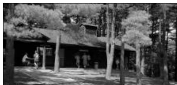
New Wall and walkway to the Horseshoe Trading Post
