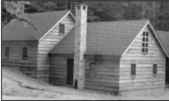
Schramm first Camp Masters' Lodge refurbished
